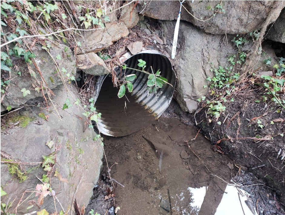
Photo 15. Piped section of Stream A under entrance to Public Works facility.
