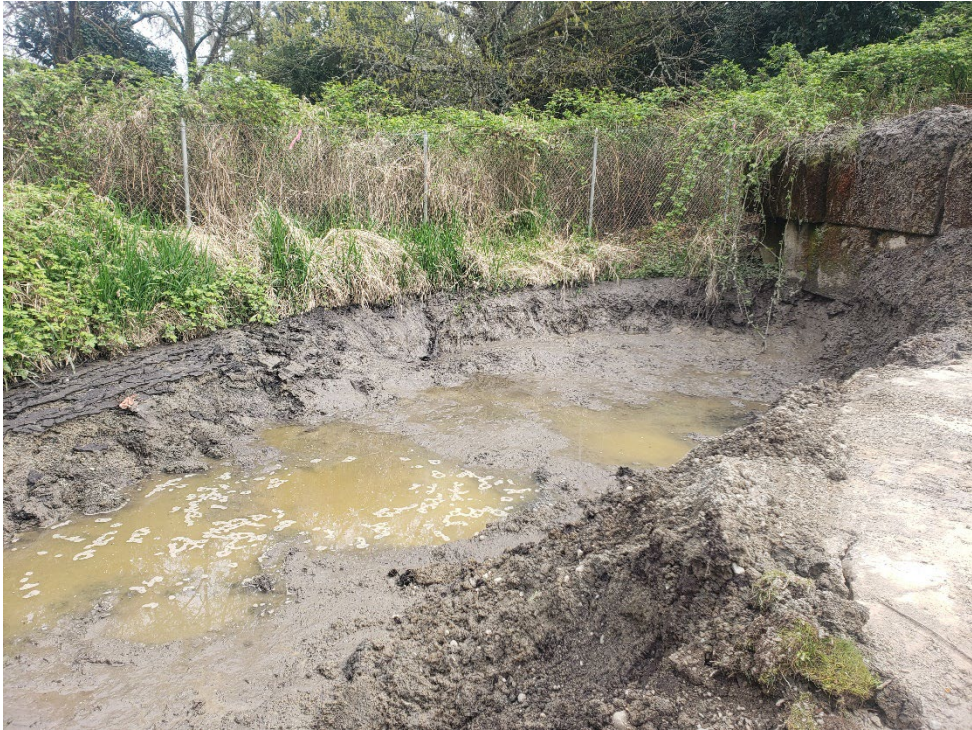
Photo 23. Stormwater feature dredged between site visits.
