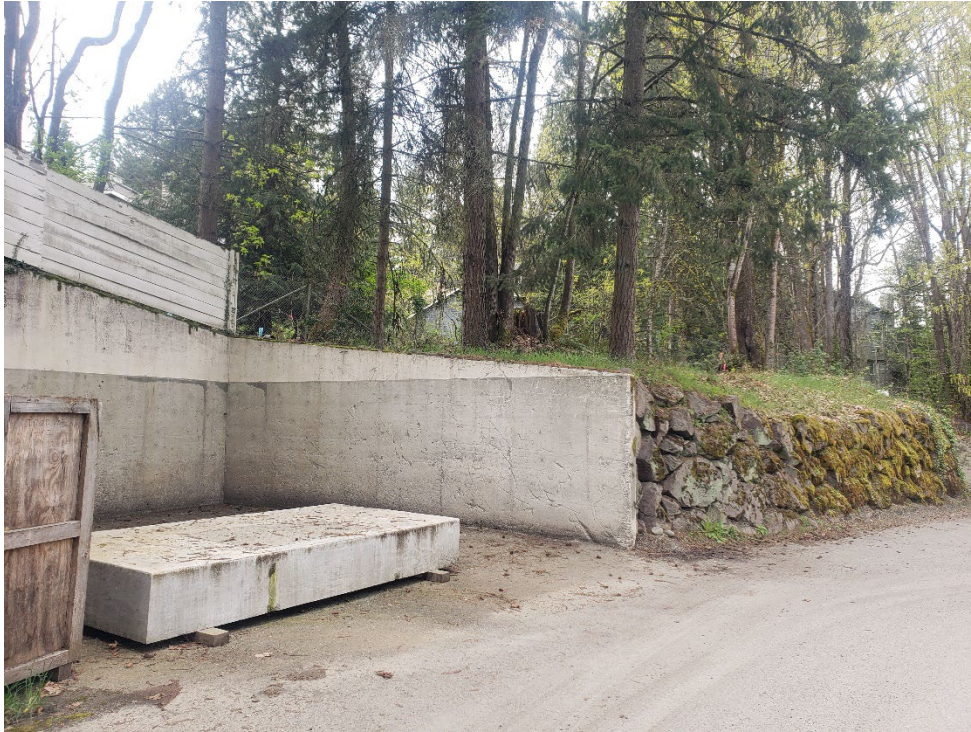
Photo 7. Perimeter of the facility contains concrete and rock retaining walls.
