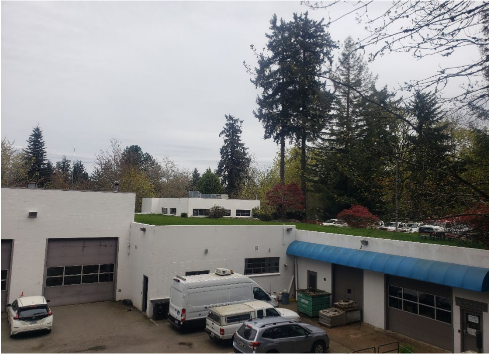
Photo 6. Public works buildings with green roofs.
