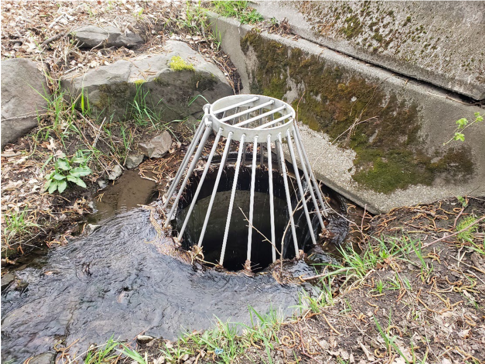
Photo 17. Stream A outlets via Type 2 catch basin (3b-221).
