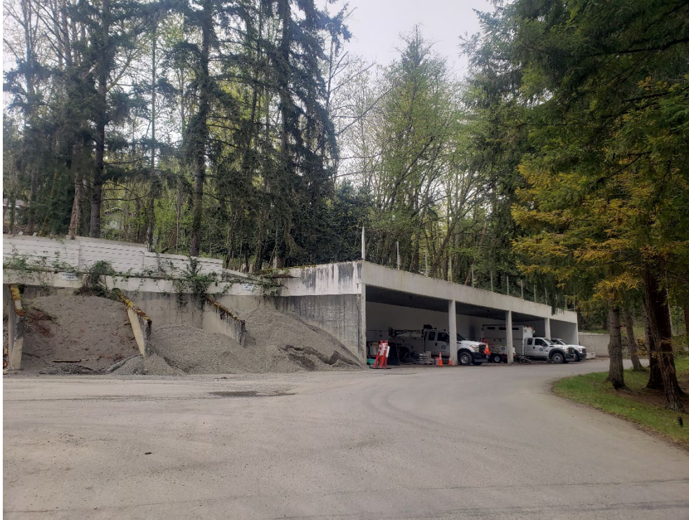
Photo 4. Concrete structures and staging areas built into forested slope.
